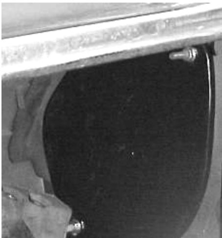
Locate in the unit box the inlet air block off.
